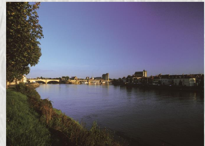
Montereau – Photo SMT ©
