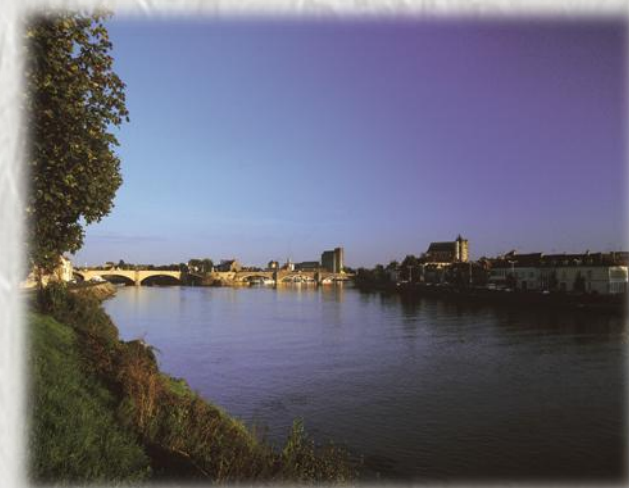
Montereau Fault Yonne – Photo SMT ©
